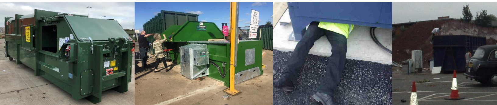
From left to right: compactor unit with a covered hopper – wastes are fed into the hopper via the opening in the side of the unit, open-top hopper compactor unit being fed by members of the public, example of too wide a gap under a compactor unit allowing crawl access to the ram, children trespassing at a HWRC site
