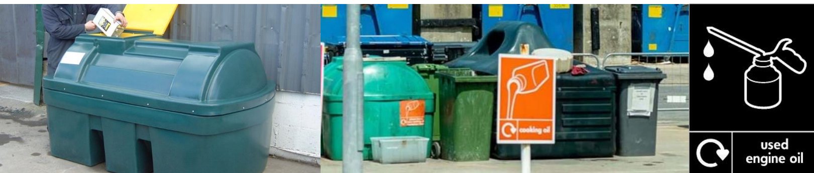
From left to right: new waste oil tank being 'road tested' (note – flammable liquid etc signage not fitted as yet), waste automotive oil and cooking oil containers with bins next to them for waste cans, bottles etc, signage
