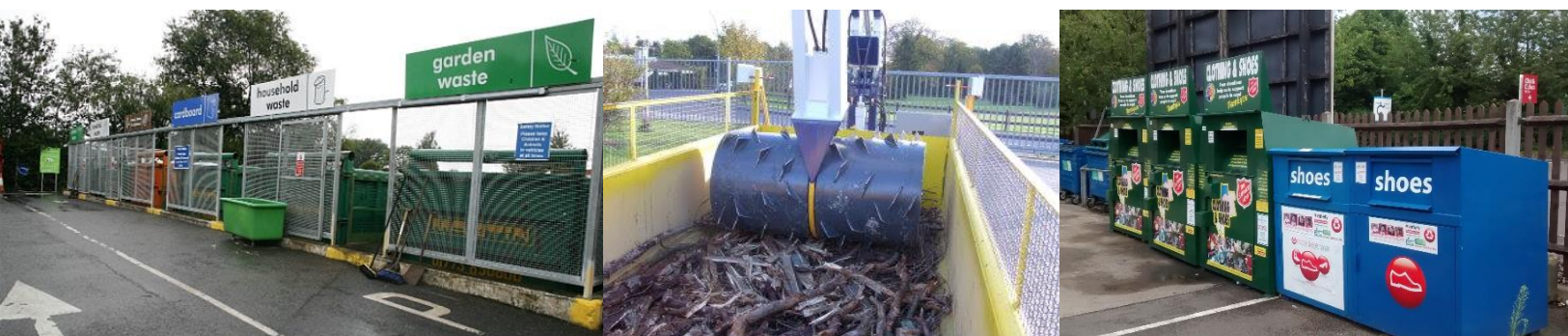
From left to right: sliding gates at a split-level site – closing the gates prevents the public loading containers during lifting, example of a roller-packer, example containers lifted by hi-ab – suitable space is required for lifting etc
